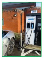
The single Rapid in Church Street car park and the 6 InstaVolt brand ones at Cobbs Farm all have both CCS (Combined Charging System) and CHAdeMo (mainly used by Nissan EVs) connectors on them but only one or the other can be used concurrently. Although they are rated at 50kW and 160kW respectively the actual rate achieved will depend on the vehicle capability and its level of charge at the time. As
